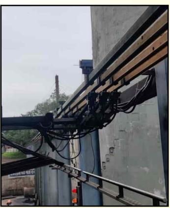
SAFE-LINE V Conductor Bar System
